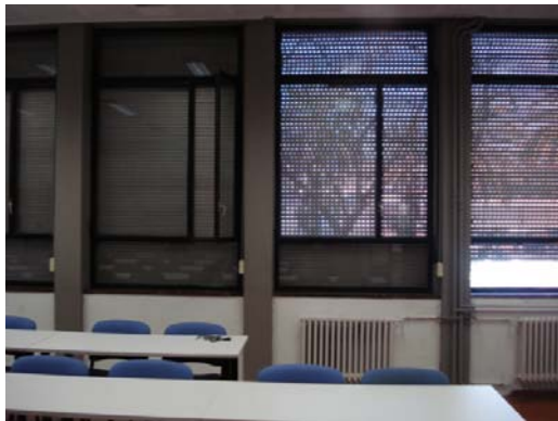
Vista interior finestres façana A
